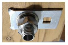
6. Install the stamped retaining washer (teeth facing up and into the plywood) followed by the flat washer, lock washer, and nut. Tighten the nut to 20 ft/lbs. using a 7/8" wrench or socket.
